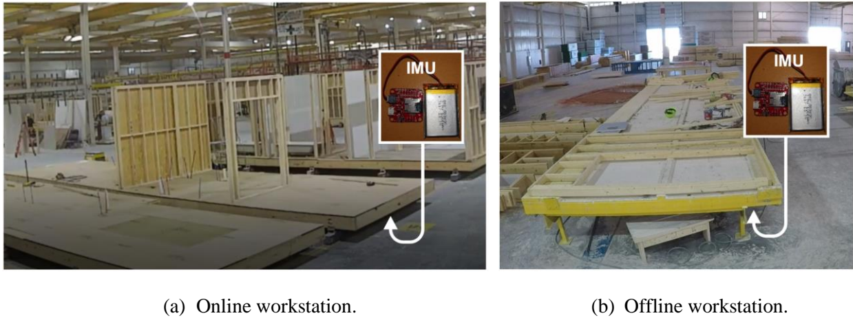
Figure 4. Location of the IMU attachment.
