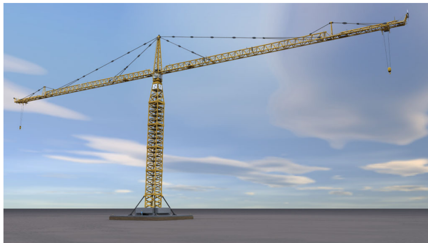
Figure 2: Tower Crane with Two Jibs
