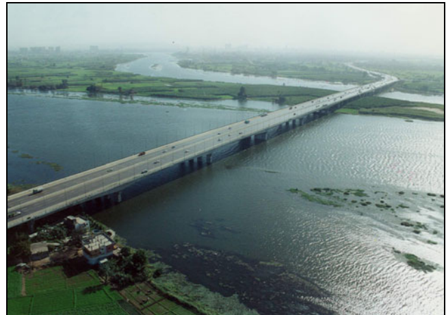
Figure 7: El-Warrak bridge after construction
