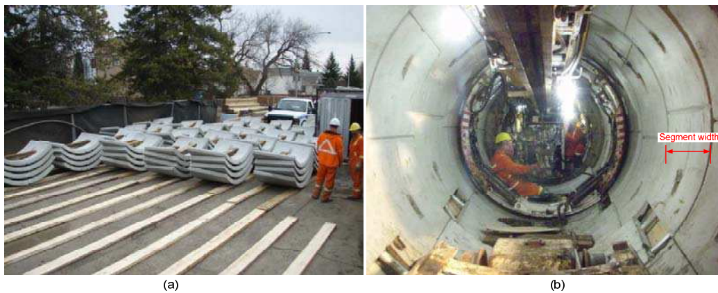
Figure 3: Segments for the project: (a) segments at the site; and (b) segments in the tunnel.
