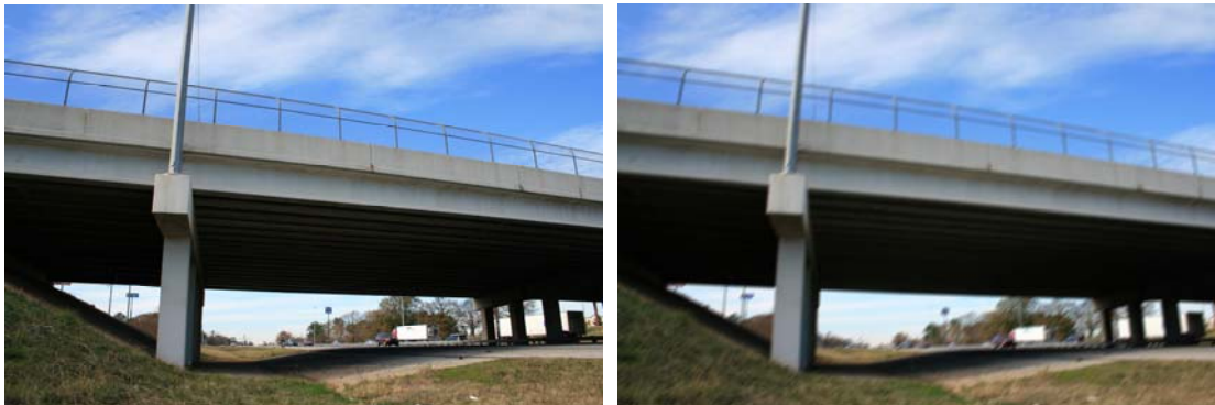
Figure 1: Comparison of two images of a bridge shot from the same position with one in good quality condition and the other distorted by a motion blur
