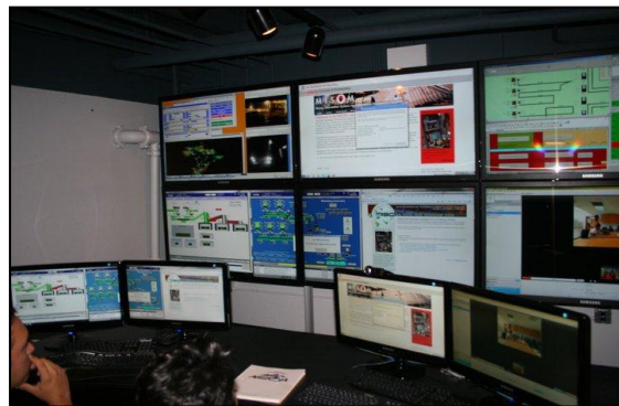
Figure 1: Control center (Nageshwaranier et al. 2011)
